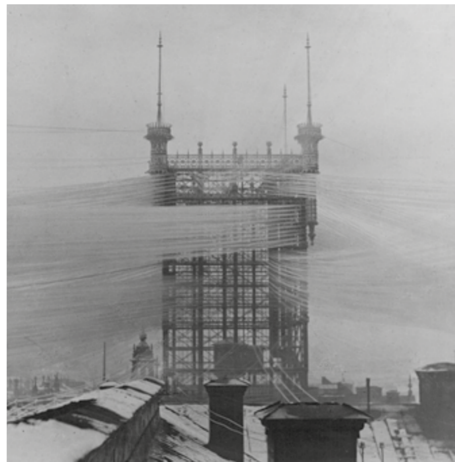
Una torre a Stoccolma collegava circa 5'000 linee telefoniche a fine Ottocento. Fonte: Wikipedia Commons. A Stockholm tower connecting 5'000 telephone lines at the end of the 19th century. Source: Wikipedia Commons.
